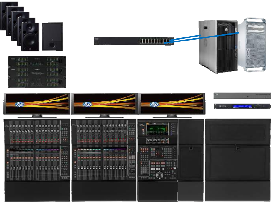
【Connection between switch and Dante Accelerator】
